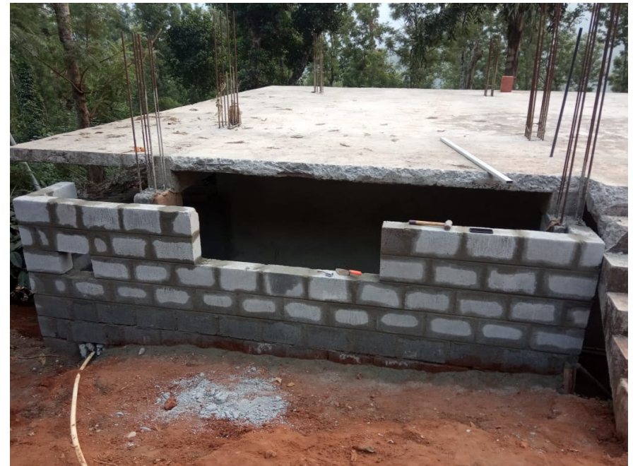
Filtration Room wall construction
