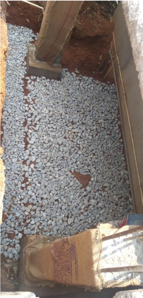
Bed soling, gravel bedding & concrete floor for filtration room
