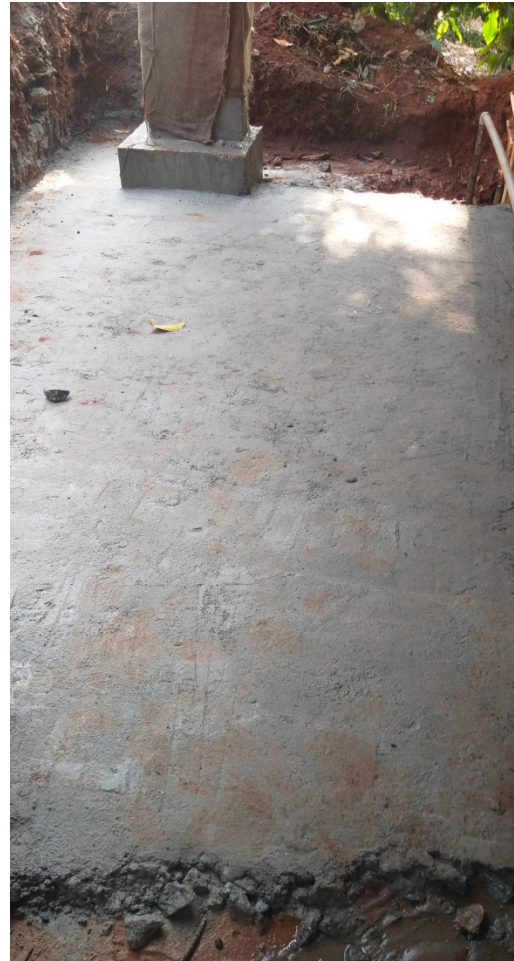
Bed soling, gravel bedding & concrete floor for filtration room
