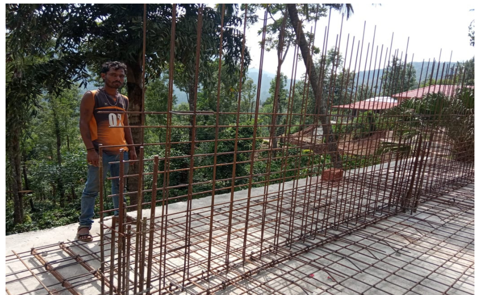
Centering for extended floor area, TMT rod bar bending for floor & wall
