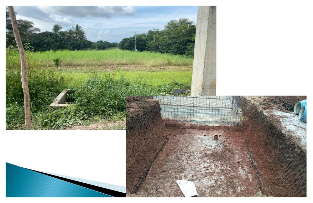
IN-GROUND SWIMMING POOL CONSTRUCTION PROJECT Plumbing work to keep main drain pipe in b/n mat of Floor Concrete & extension up to filtration room
