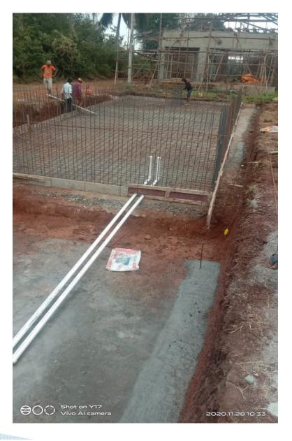
IN-GROUND SWIMMING POOL CONSTRUCTION PROJECT Floor Concrete work, Fixing of Skimmer Boxes, Pipes for pool filtration fittings and mat preparation for pool concrete wall.
